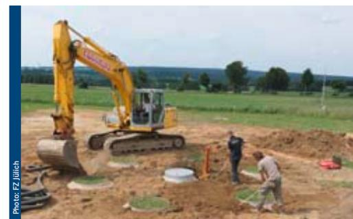
Six additional lysimeters are set up in a circle around every central measurement- and service shaft (top) Once the lysimeters have been set in place and the technology has been installed, the surrounding pit is filled in with soil (bottom)
